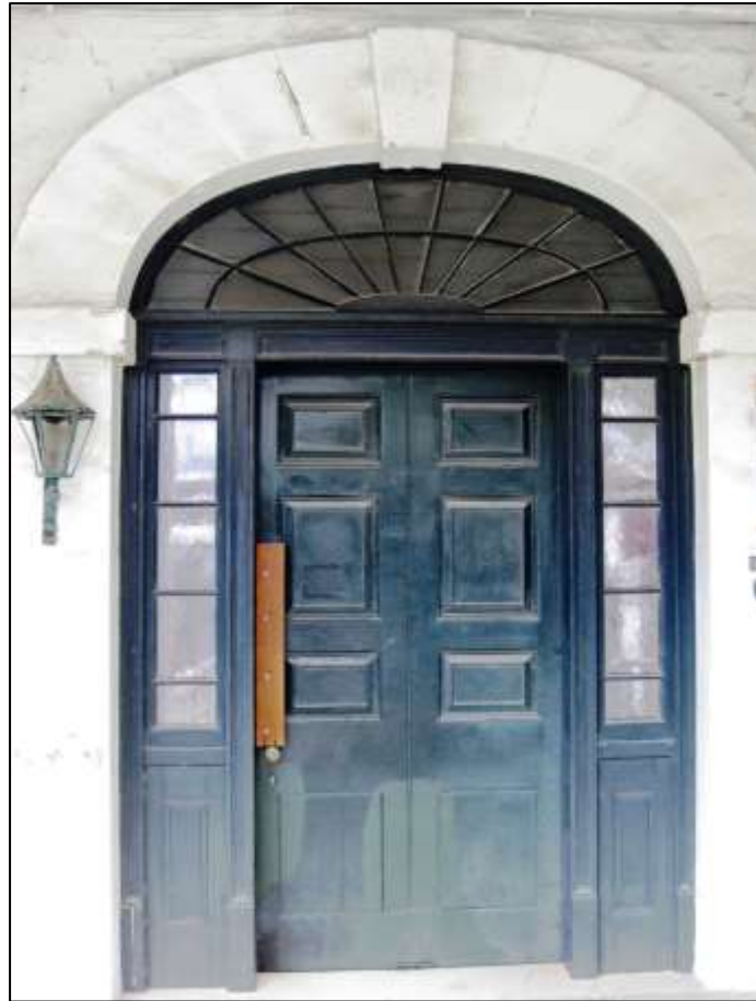
Figure 2 Cleveland House front door
